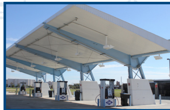
City of Bossier: CNG Fueling Facility.
